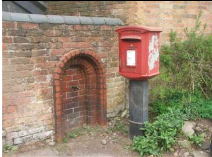
Figure 26 Wall and post box in front of village shop
