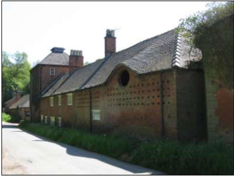
Figure 21 Swynnerton Hall barns – The roof covering of Staffordshire blue clay tiles probably replaced thatch.
