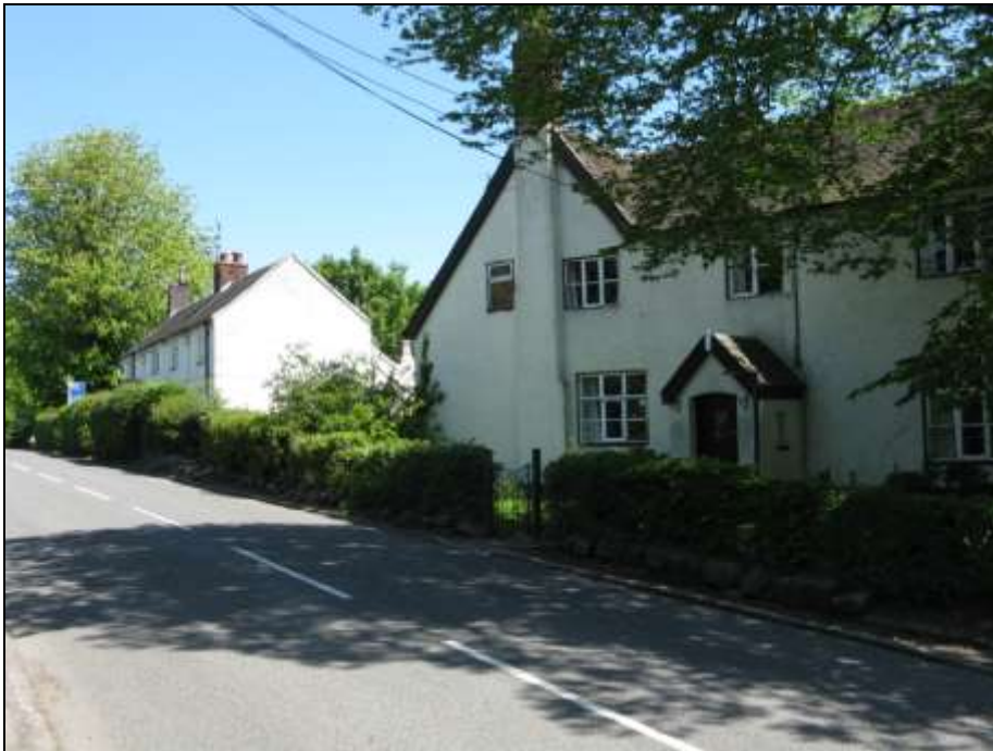
Figure17 Gable orientations add interest to linear cottages along Main Road
