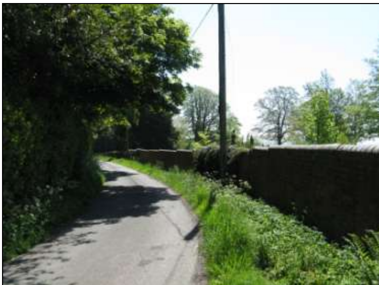
Figure 31 Estate Boundary wall to Swynnerton Hall
