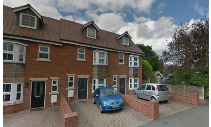
No soft landscaping to front of the properties making car parking the dominating feature to the frontage
