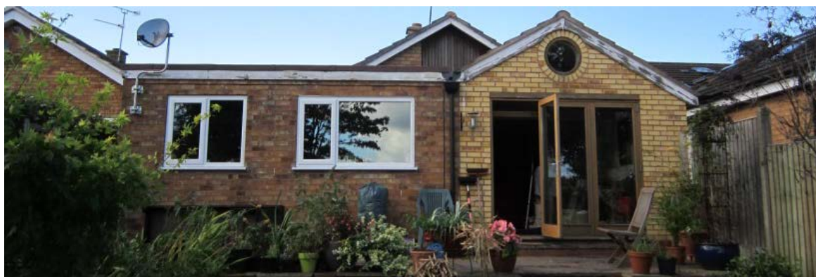
An example of piecemeal rear extensions to a bungalow which detract the property
