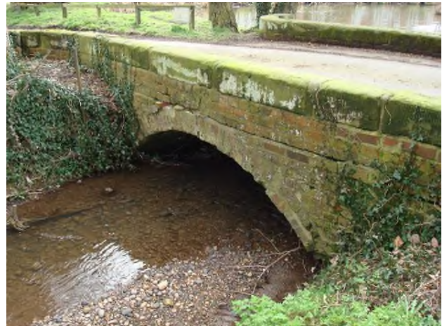
Figure 5: The bridge adjacent to the site
