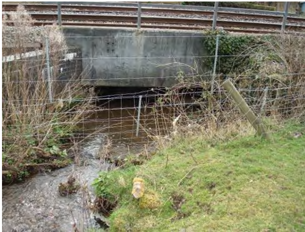
Figure 4: The culvert in which the Jolpool Brook flows under the railway
