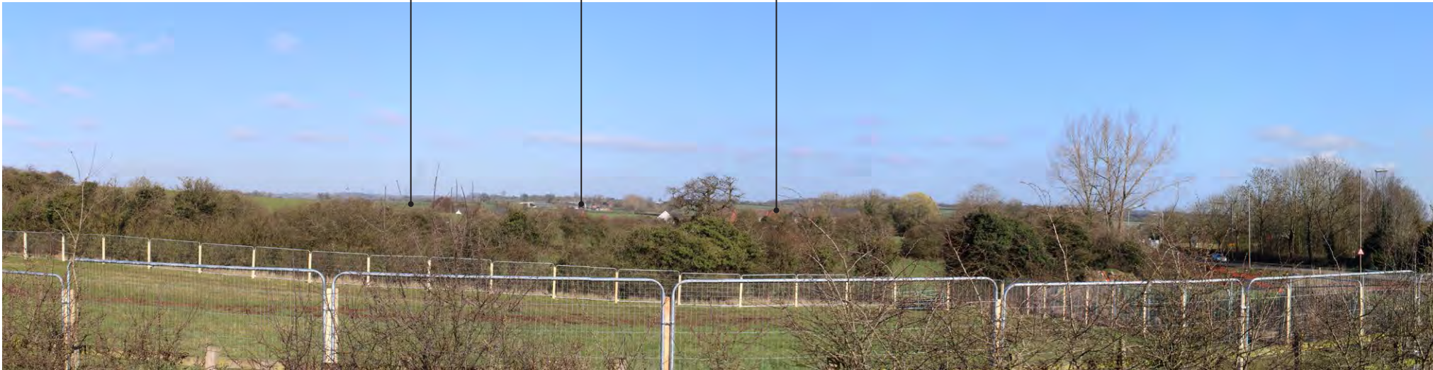
View from Quincy Way looking north east towards the Site Photograph 29
