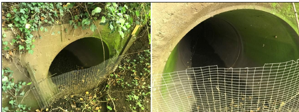
Figure 4: Culvert immediately upstream of Marston Lane
