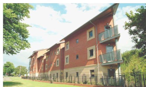
Bournbrook Court Birmingham 35 Apartments
