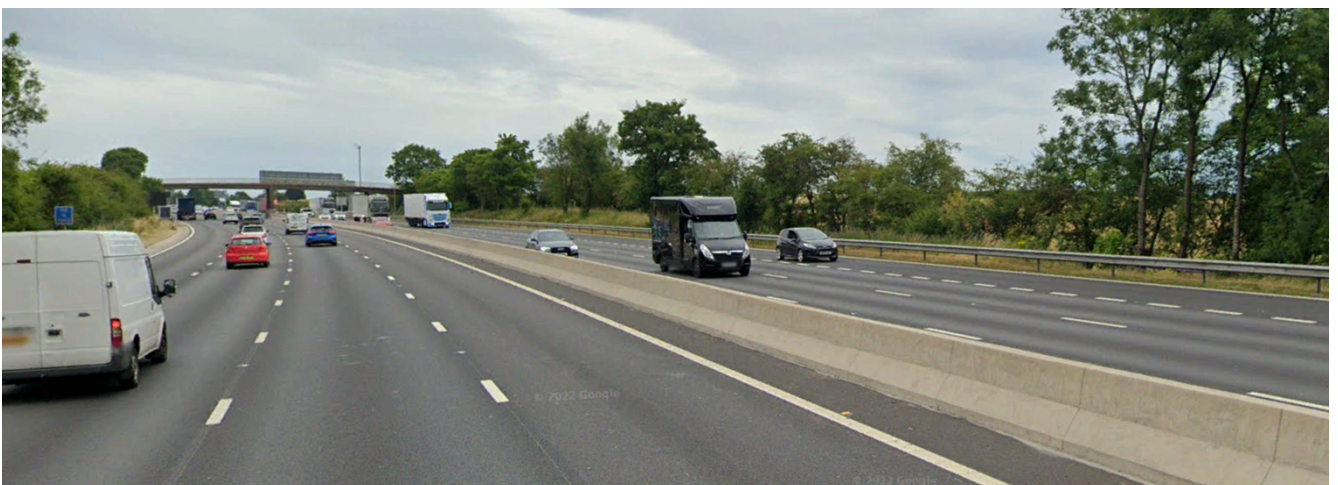
View F. M6 travelling north. Google earth screen snapshot.
