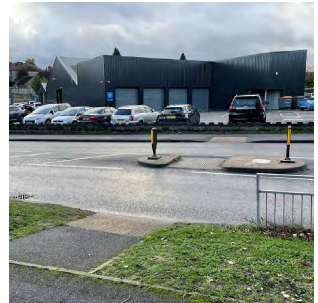
Toucan Crossing on Milford Road to The Rise
