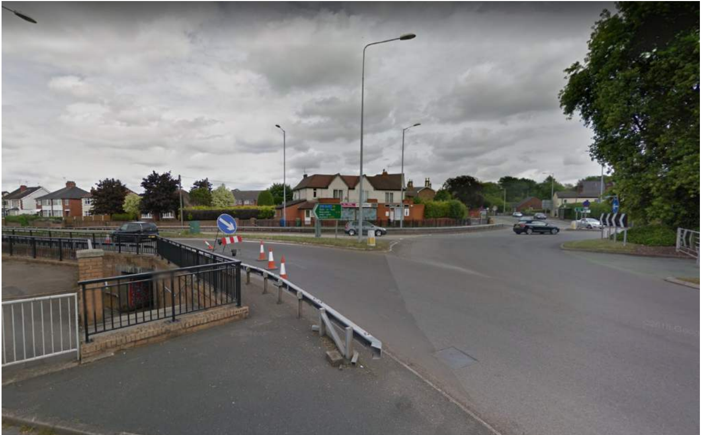
Figure 3.1 Extract from Google Street View (2022) Showing Pedestrian Underpass
