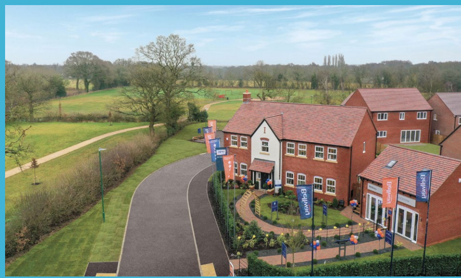
Photograph of Bellway Development at Tidbury Heights incorporating a new country park
