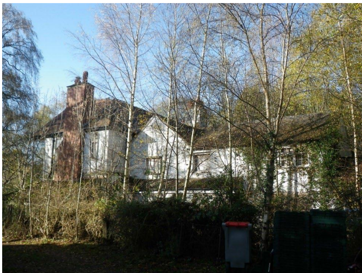
Figure EDP A2.20: The abandoned house (south-eastern elevation).
