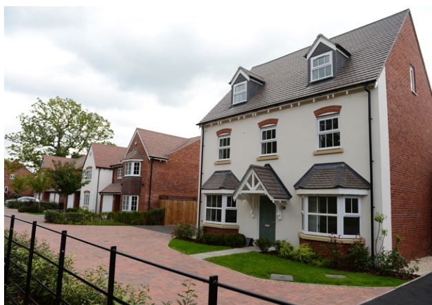
Photograph of Bellway Development at Dickens Manor
