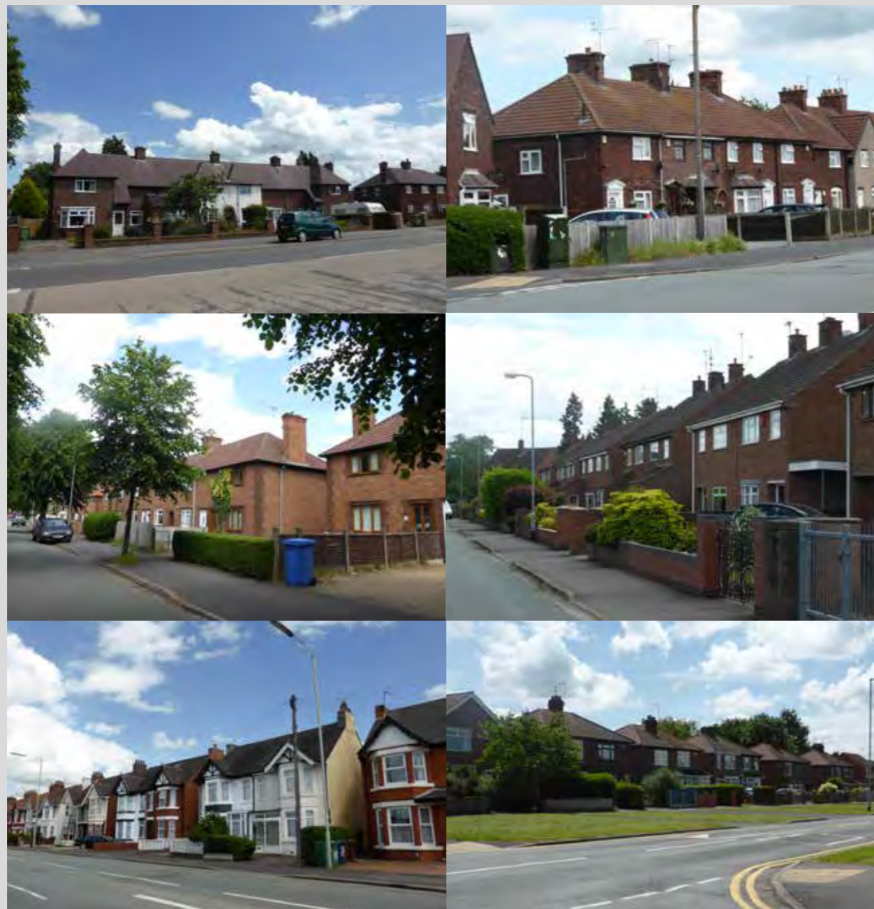
1920's development of semi-detached and terraced properties with ginnels in red brick with concrete tiled roof. 5 to 6 metre front gardens, on street parking with some retro fitted on plot parking. Perimeter block layout
