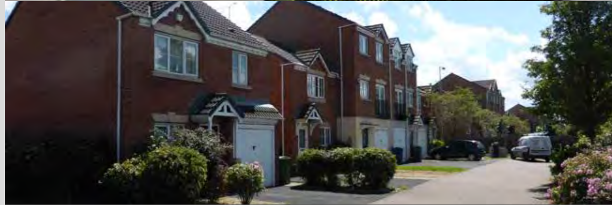
Modern infill development of 2 and 3 storey town houses with integral garages and parking to the fronts of properties. Feature Juliet balconies and gables above top floor windows. Hard surfaces dominate the public realm.
