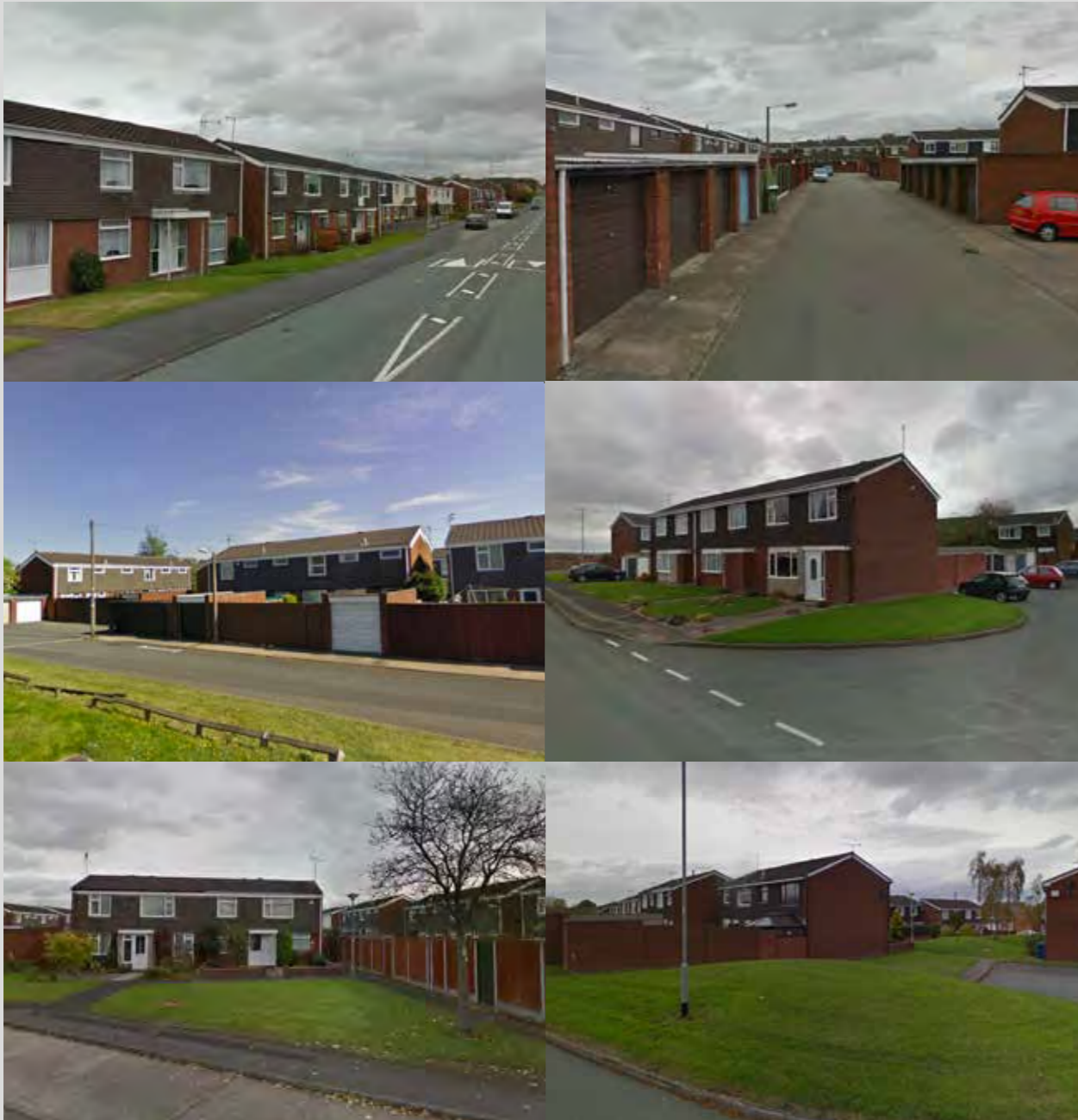
Radburn style terraced development fronting onto open spaces. Vehicular access only to rear parking courts. Red brick construction with tile hanging to front elevation. Low pitched tiled roofs with end gables. Well connected communal open spaces throughout the development separating pedestrians from vehicles.
