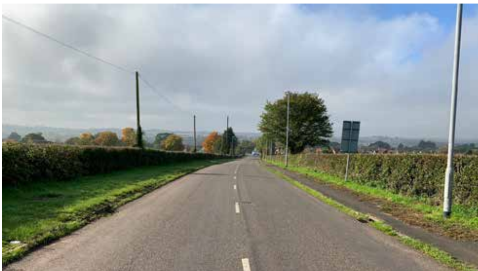
Uttoxeter Road along the site frontage
