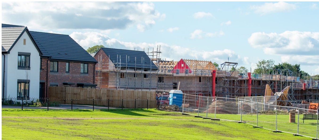
Houses under construction locally
