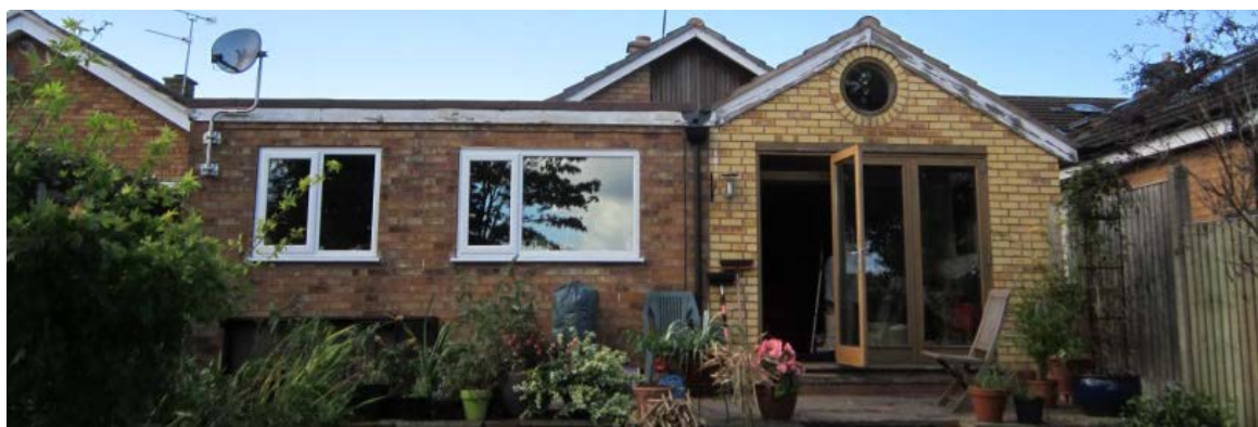
An example of piecemeal rear extensions to a bungalow which detract the property
