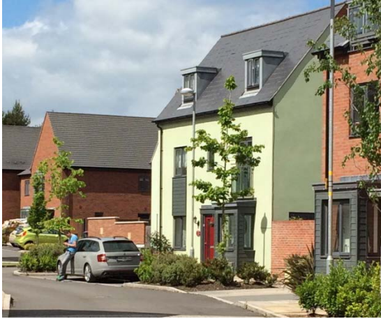
Car parking to front of properties broken up with soft landscaping
