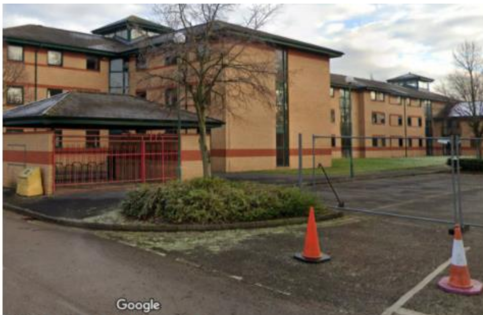
Stafford Court Beaconside Stafford. From Google
