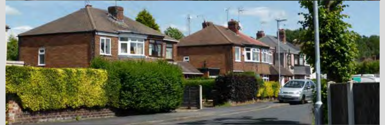
Post war semi detached and terraces. Red brick concrete tiled roofs. Hipped roofs. 5 to 6m front gardens some converted to parking.
