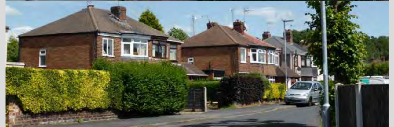
Post war semi detached and terraces. Red brick concrete tiled roofs. Hipped roofs. 5 to 6m front gardens some converted to parking.
