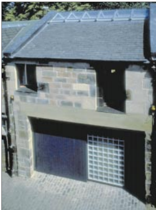
THE UNDIVIDED GROUND FLOOR SPACES IN MEWS BUILDINGS MAKE THEM EASY TO ADAPT. SUCH FLEXIBILITY CAN BE DESIGNED INTO NEW BUILDINGS ▲
