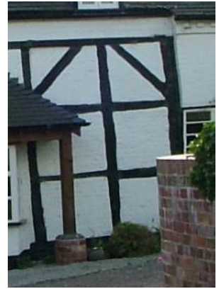
Timber Framing with Brick Infill Panels
