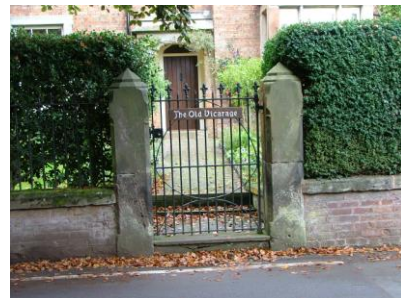
Stone gate piers and cast iron gate at The Vicarage
