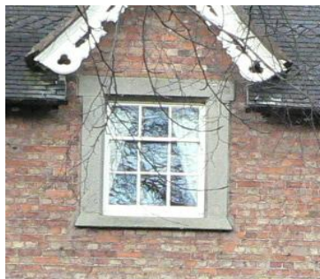
Three-over-six sash window at the Old Vicarage
