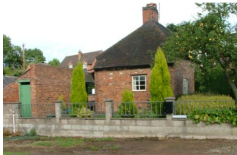
Concrete wall and steel fence to Spring Farmhouse
