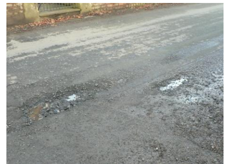
Damage to Wall from road salt Pitted road surface on Church Lane
