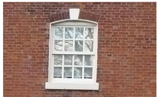
Eight-over-eight sash window at Church Farm
