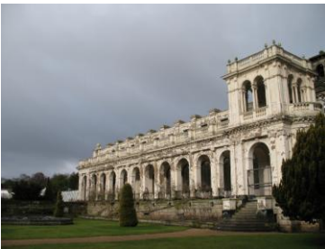
South Elevation of Former Service Block
