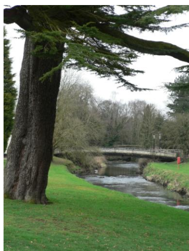
1930s Bridge on site of former Iron Bridge
