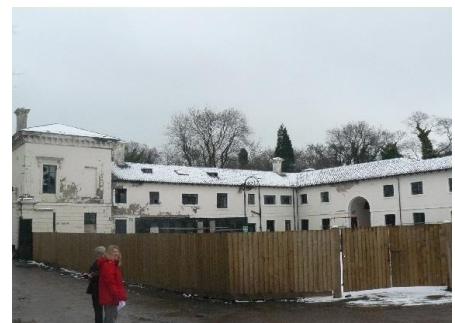
Stable Block and Rear Courtyard
