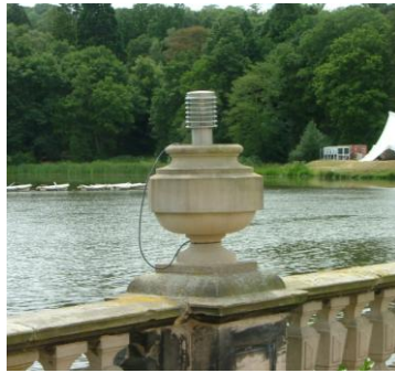
Replacement Urn with Intrusive Modern Lighting
