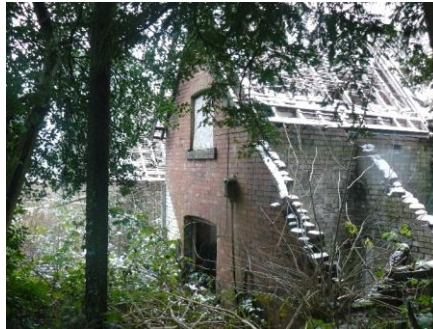
1-4 Park Drive, a Derelict Listed Building
