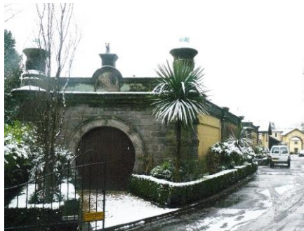
Former Smithy with Rear Access Road
