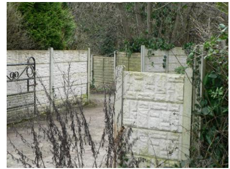
Intrusive Concrete Fencing
