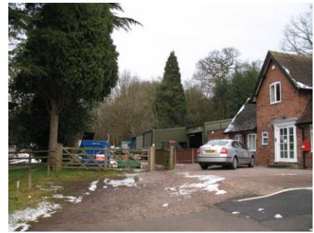
Golf Club Offices and Maintenance Building
