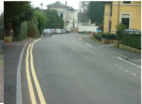
Road markings to Park Drive
