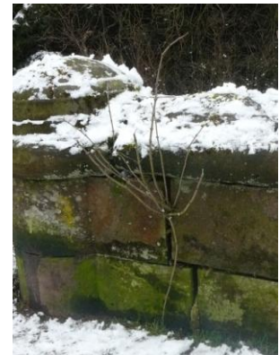
Condition of Bridge
