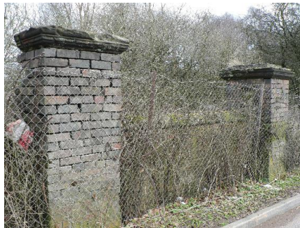
Part of Wall near Knowle Wall Farm
