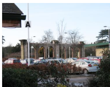
Remains of Ballroom Arches Incorporated into Car Park
