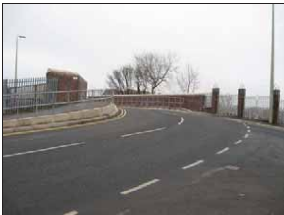
Doxey Road Railway Bridge
